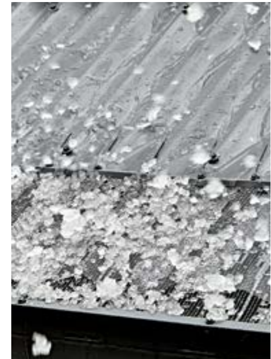
2mm Steel Gutter Mesh installed
